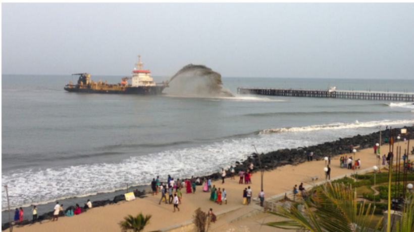
Dredger spewing sand towards the Pondy shore
