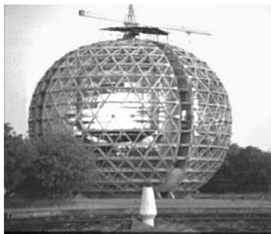
The outer space frame is in place
