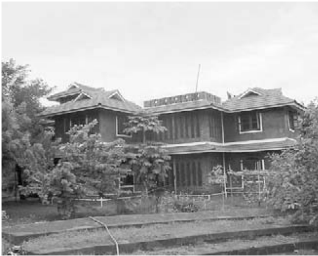
The Adishakti guest house. The inner walls are brick, the outer walls are of golden brown mud; traditional experts in this kind of construction were specially called, experiments made to check for strength before the technology was finally used. Interestingly a bushy plant which keeps snakes away (and is also an antidote) lines the entrance.
